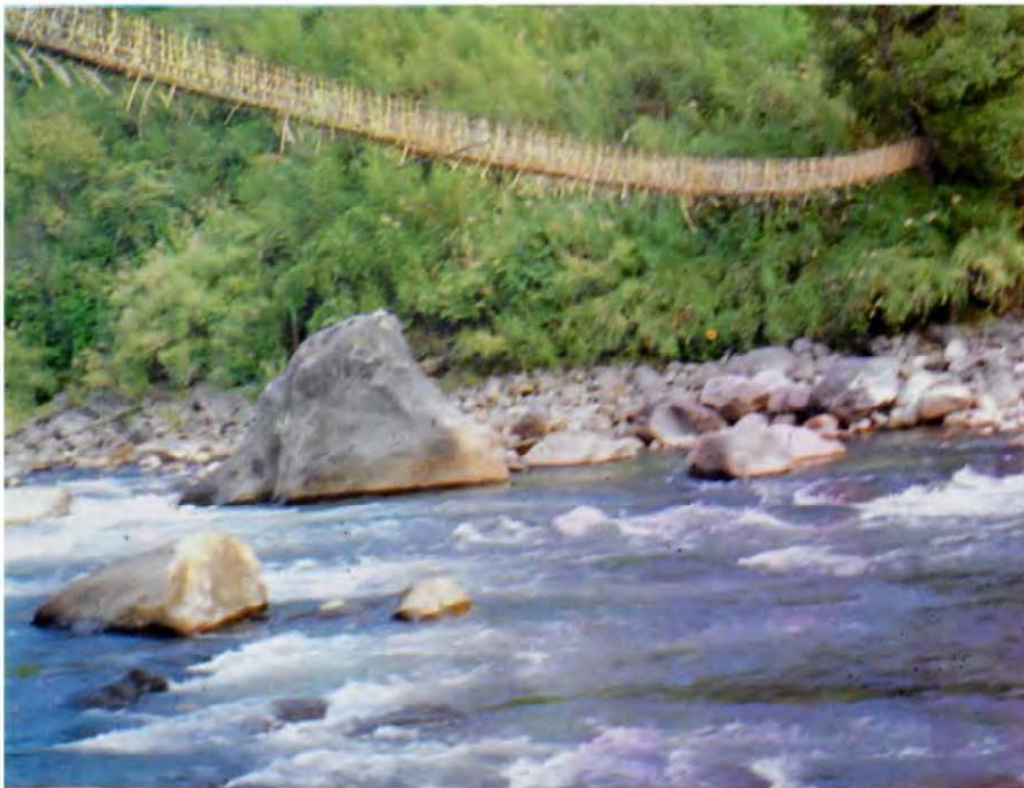
Dibang Valley - A typical hanging bridge made of canes, bamboos and liana on a river. (Courtesy : Manas Bhaumik & M.K. Pathak)
